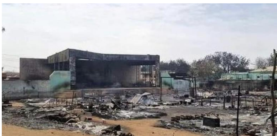
Image: The Performing Arts Theatre in el Geneina after the destruction
